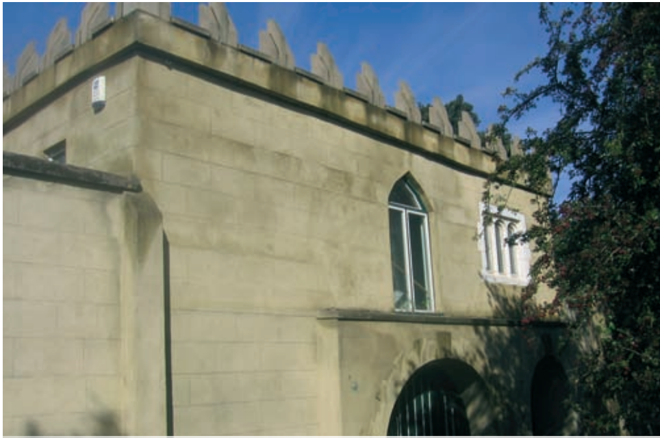
The Bothy, a grade II listed structure which forms part of the Avenue House Estate
